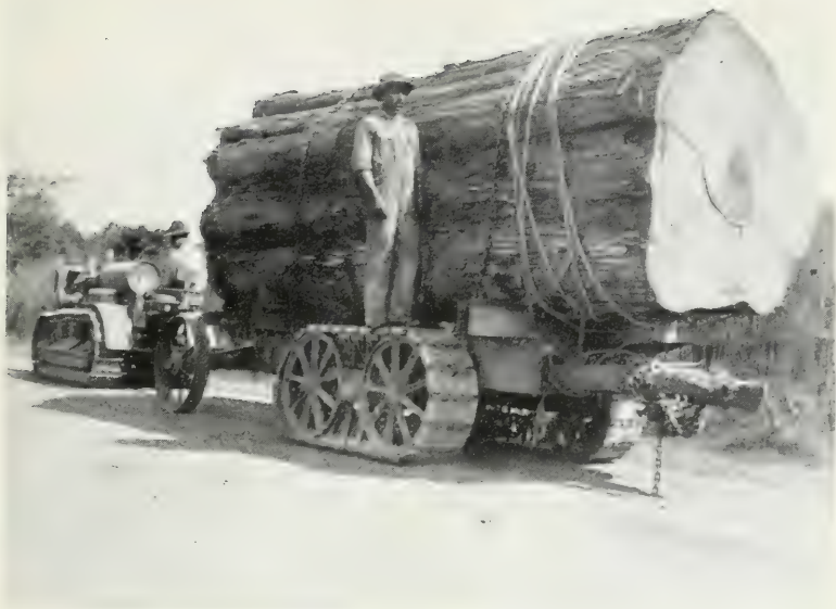
FIG. 137. CATERPILLAR HAULING 1100-YEAR-OLD CYPRESS LOG ON 19 MILE HAUL, U.S.A.
